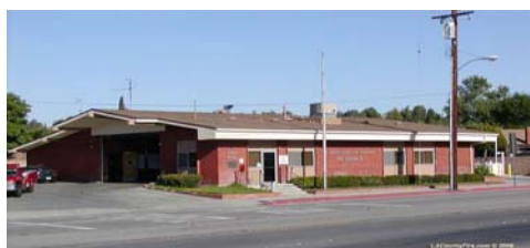
Los Angeles County FD Station 111
